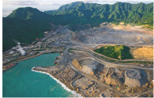
Fig. 4 Lihir Gold Mine and its power supply
