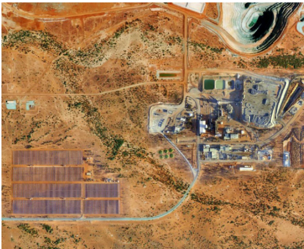
Fig. 1 Degrussa Mine with its power supply
